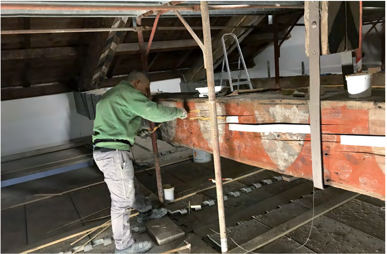
The wooden trusses were consolidated and restored using products from the MAPEWOOD SYSTEM (MAPEWOOD PRIMER 100 and MAPEWOOD PASTE 140).
