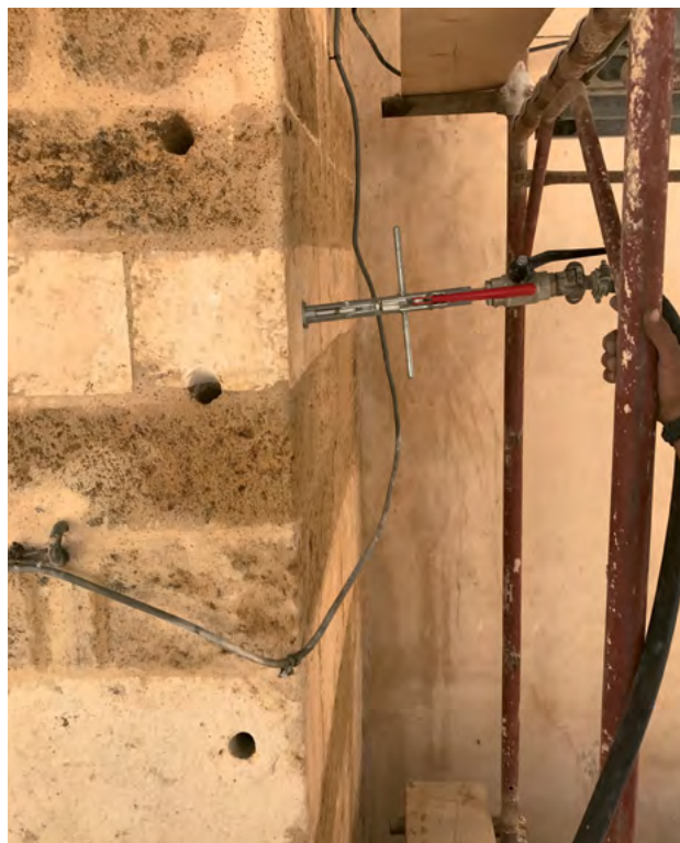
MAPE ANTIQUÉ F21 super-fluid binder was injected through small tubes using low-pressure pumps to consolidate the stone structure.
