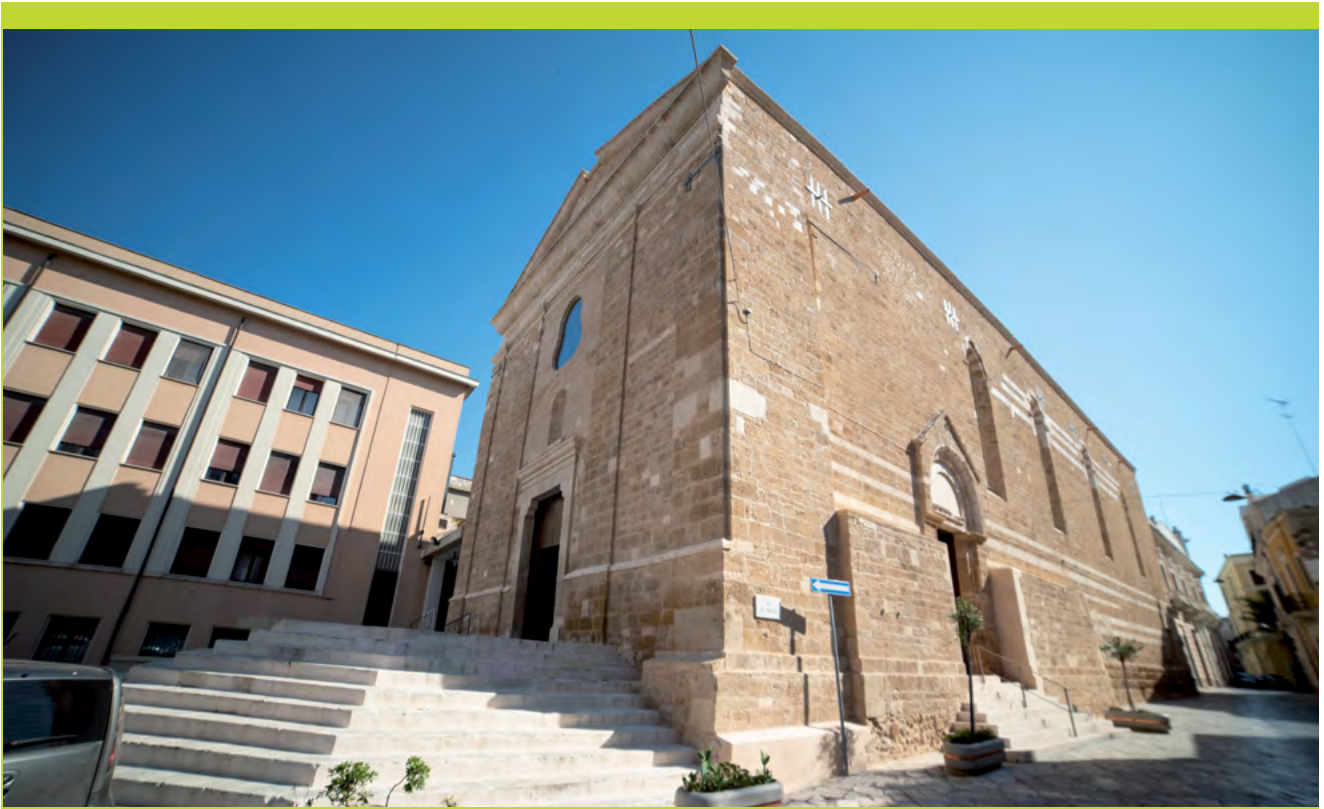
Built in the 14th century, the Church of San Paolo Eremita recently underwent structural strengthening and renovation of the masonry.
