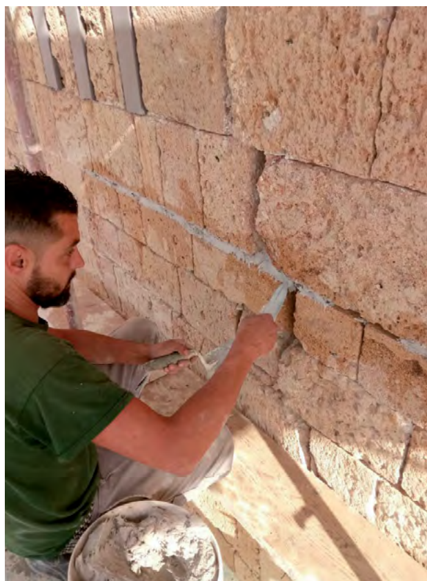
For the installation layers and for pointing of the 'natural finish' masonry of the church, the product chosen was MAPE-ANTIQUÉ ALLETTAMENTO salt-resistant masonry mortar, made from natural hydraulic lime and Eco-Pozzolan.
