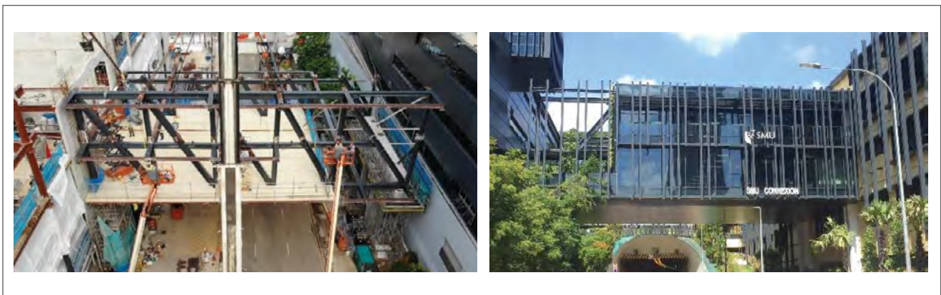
Modified Pratt trusses to support the two-storey link building.
