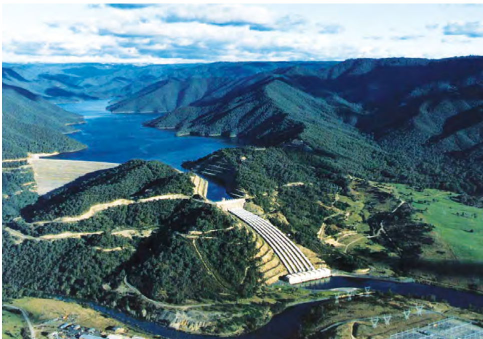
SMEC, a member of Surbana Jurong Group, is involved in Snowy 2.0, the expansion of the Snowy Mountains Hydro-electric Scheme which is recognised as one of the seven civil engineering wonders of the modern world. SMEC contributed to the technical and financial feasibility of the project and has been engaged as the 'Owner's Engineer', providing technical advice and engineering support to help deliver this innovative renewable energy project. The project, which is currently under construction, involves the linking of the two existing reservoirs of Tantangara and Talbingo, through approximately 27 km of underground power waterway tunnels. There will also be a new underground power station with pumping capabilities.
