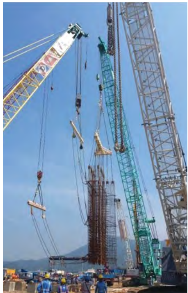
Figure 13: Y-panel rebar cage lifting operation.
