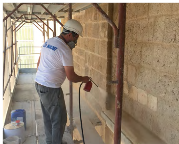
The stone surfaces of the church were protected from the action of rain with ANTIPLUVIOL W water-repellent impregnator.
