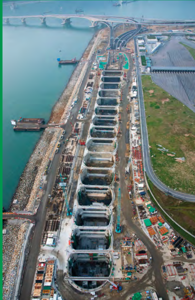
The 15-cell caterpillar-shaped cofferdam.
